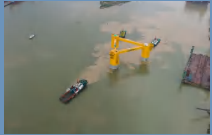
"FUYAO" departs Dongguan Yard prior to installation
