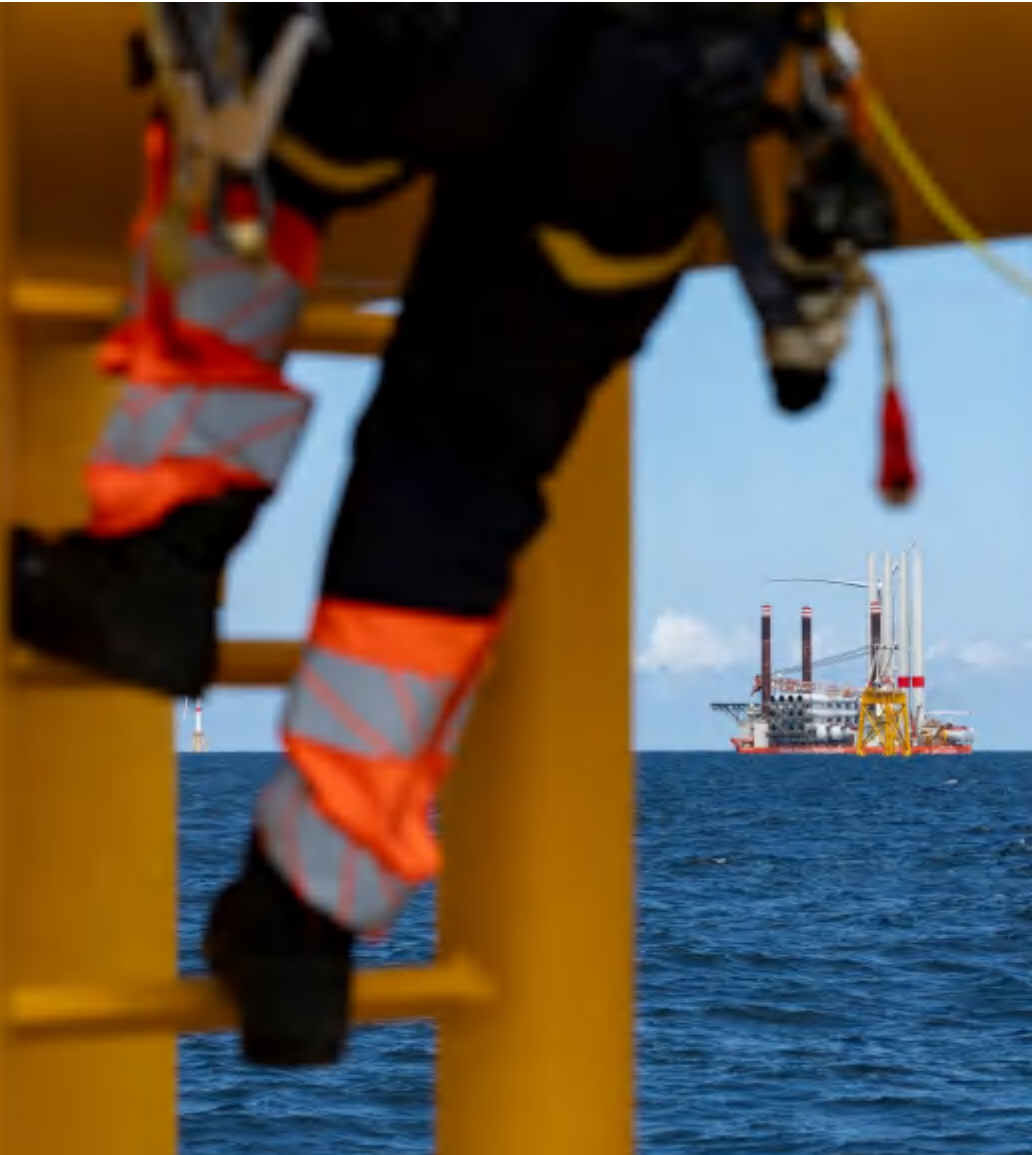
A technician accesses a foundation / Saint Brieuc Windfarm -France – C.Beyssier
